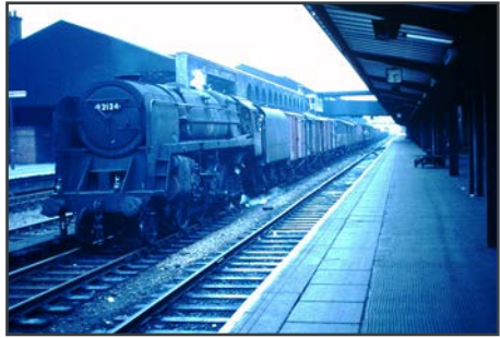
BR class 9F 2-10-0 92124 passes through Chester station on 4th July 1966 with a freight to Birkenhead. These were the largest locomotives to work on the network, apart from the relatively small number of Beyer Garratts and, towards the end of steam the class was synonymous with Birkenhead locomotive depot, it having in the region of fifty allocated there. (©John Cashen)
