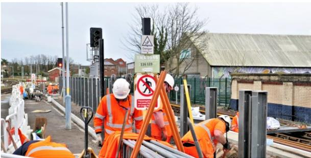
*Southport station- Posts (grey) being erected for a barrier to separate off the end of platform 1*
